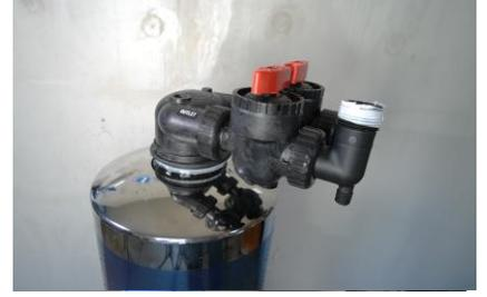
Disconnect the carbon filter tank from the system
