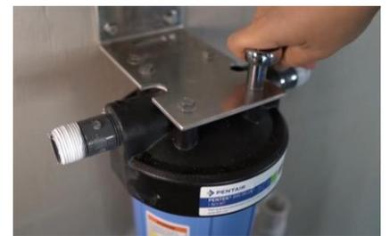
32) Use the remaining 4 bolts to secure the sediment filter to the mounting bracket.
