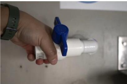
36) It is suggested to connect a PVC shut off valve onto the threaded adapter from the incoming water supply. Ensure it is fully tightened.
