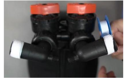
39) Apply plumbers' tape to the inlet and outlet connections on the carbon filter tank.
