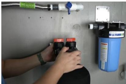
40) Position the carbon filter tanks next to the sediment filter. Ensure the connections on the tank are facing backwards against the wall.
