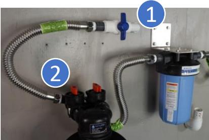
48) Ensure the shut off valve to the system is closed (1), and that the bypass valves on the carbon filter tank is set to bypass (2). Turn the water back onto the home and inspect the shut off valve for leaks.
