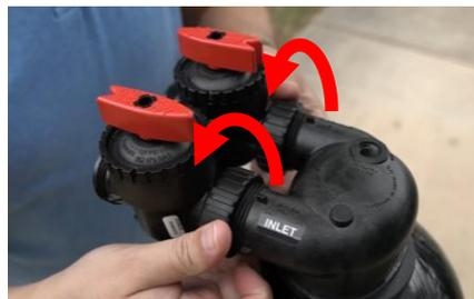
11) Fully tighten the fasteners on both valve connections securing the bypass valves.
