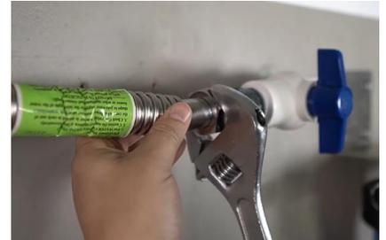
38) Connect a corrugated pipe to the PVC nipple. Ensure it is fully tightened.
