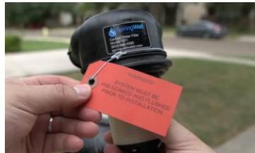
3) Locate the tank head and note the label discussing the necessary 48-hour pre-soak.
