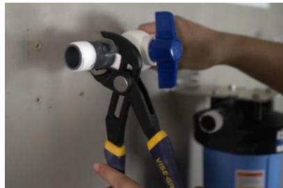
37) Connect a PVC nipple to the other end of the PVC shut off valve. Ensure it is fully tightened.
