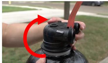
6) Turn the tank head clockwise until it is fully tightened.
