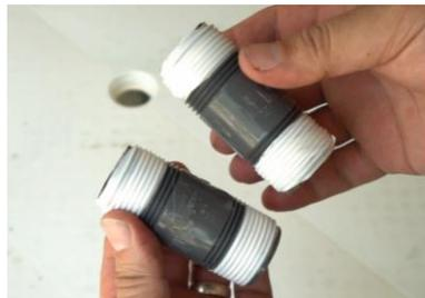
27) Note: Plumbers tape will need to be applied to all PVC threads during the installation.
