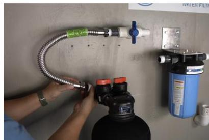
41) Connect the corrugated pipe from the shut off valve to the inlet on the Carbon filter tank. Ensure it is fully tightened.
