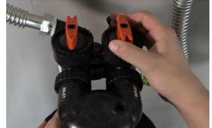
50) If no leaks are detected, open the bypass valve to allow water flow through the tank.
