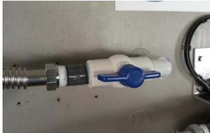
49) If no leaks are detected, open the shut off valve and allow water to flow through the system. Check the connections for leaks.
