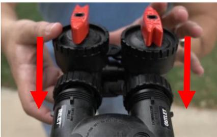
10) Insert the bypass valve onto the connections of the tank head and press in place.
