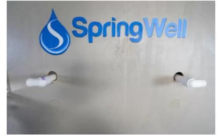
33) Expose the pre-plumb and prep to connect the system. Threaded adapters are used in this example.
