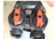
Bypass off, water flows through tank
