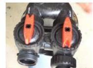
Bypass off, water flows through tank
