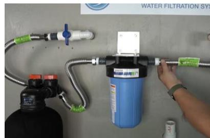
44) Connect a third corrugated pipe to the outlet from the sediment filter. Ensure it is fully tightened.
