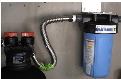
43) Connect the other end of that corrugated pipe to the inlet side of the sediment filter. Ensure it is fully tightened.
