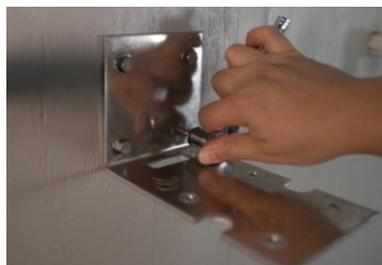
30) Use a 3/16" drill bit to pre-drill the holes for the sediment filter mounting bracket. Use 4 of the provided bolts and washers to secure the bracket to the wall using a 1/2" socket.
