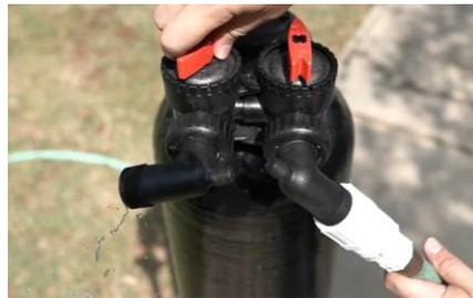
17) Switch off the bypass on the tank. Note: Some water may be released from the 48-hour pre-soak.
