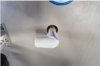
34) 1" threaded adapters are featured in this guide and are installed on the incoming water supply with the threads towards the location of the carbon tank.
