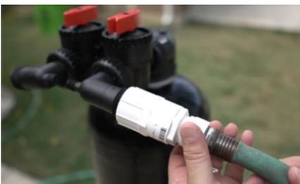
13) Use the hose bib to attach the lawn hose to the inlet on the first tank. Ensure the bypass is off to allow water flow through the tank.
