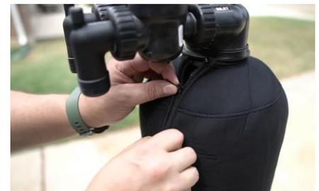
Note: The neoprene jacket that was shipped with the tank can now be zipped onto the tank. The Springwell logos should face forward.
