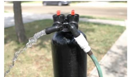
18) Turn on the water and allow the tank to flush for about 3-5 min. Until the water runs clear.
