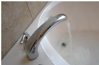
51) Allow water to run through the system for 5-10 minutes. It is normal to see a small amount of sediment during this time.
