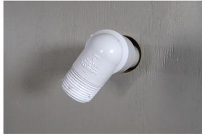
35) Point the threaded adapter for the opposite end of the pre-plumb towards sediment filter outlet connection.
