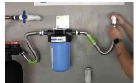
45) The other end of that corrugated pipe will be connected to the pre-plumb that leads into the home.
