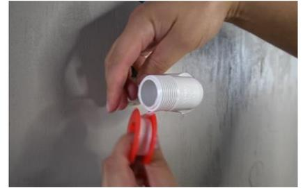
**NOTE:** Plumbers tape will need to be applied to every thread when connecting all corrugated pipes.
