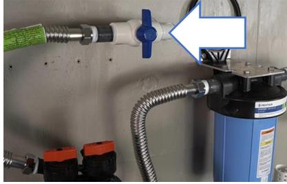
Turn the shut off valve to the off position.
