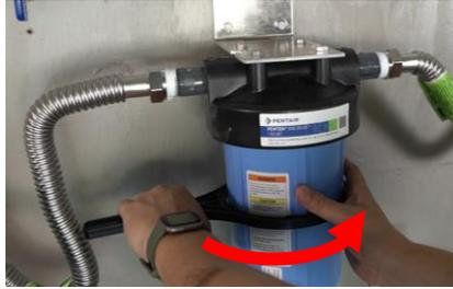
46) Before turning the water back on to the home, use the provided spanner wrench to fully tighten the sediment filter housing.
