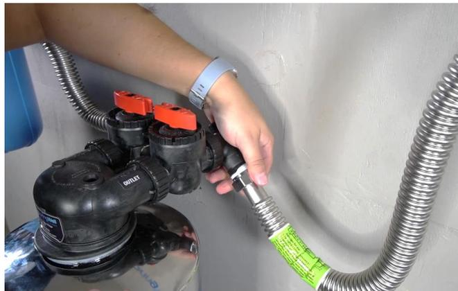
Reconnect the tank to the system and proceed back to page 11 to test the system again.
