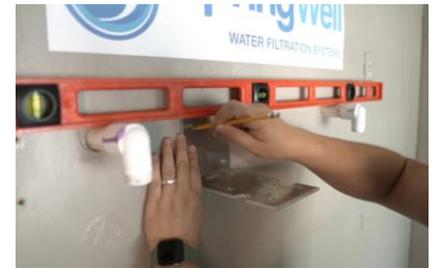
29) Identify the optimal area to mount the sediment filter. Ensure that it aligns to allow room for the carbon filter tank ahead of the sediment filter. Also note that the distance from the outlet of the sediment filter is close enough to the pre-plumb. Mark your holes for pre-drilling.
