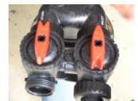
Bypass off, water flows through tank
