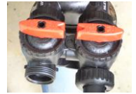
Bypass on, water does not flow through tank
